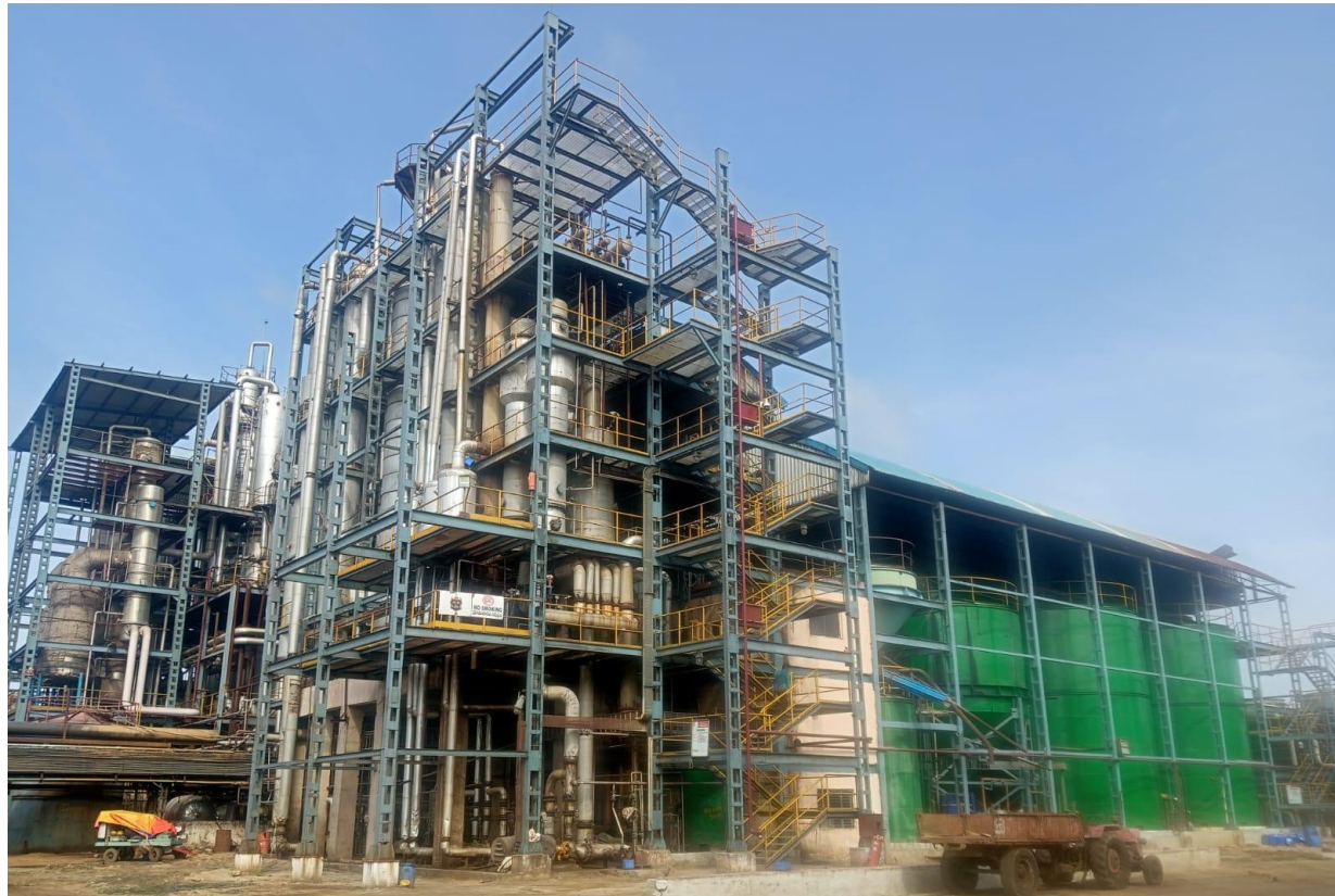
Picture 4: The Evaporation and DDGS dryer sections of Distillery unit
