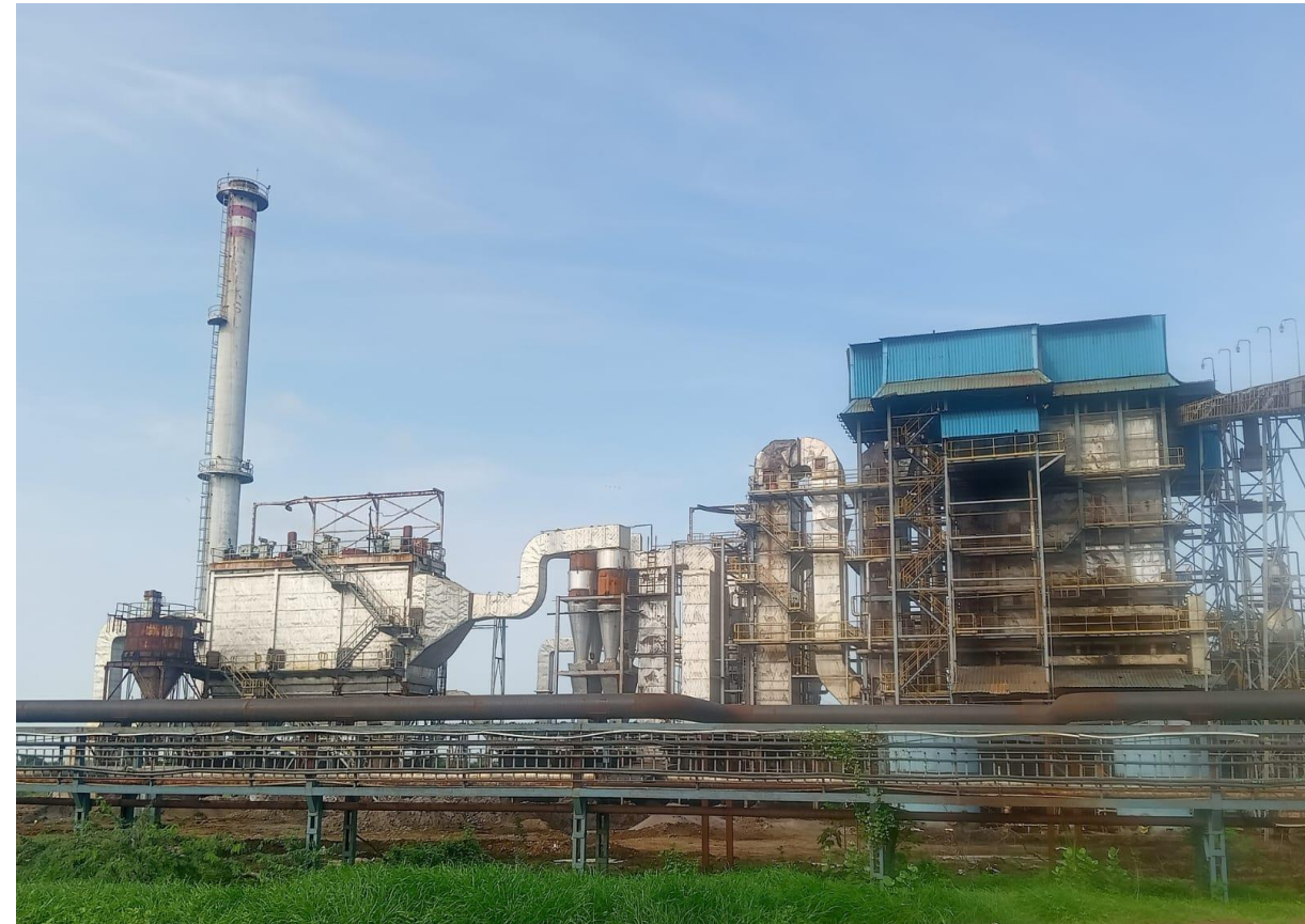
Picture 3: Boiler, ESP and chimney sections of the co-gen unit
