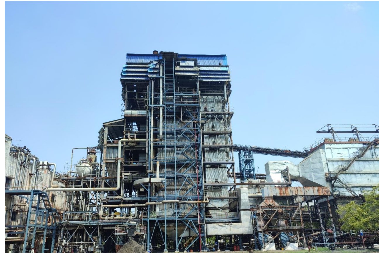
Picture 3: Boiler, ESP and chimney sections of the co-gen unit
